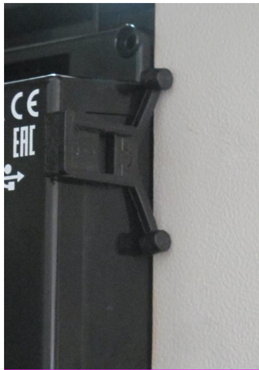
Installation of self-retaining type bracket
